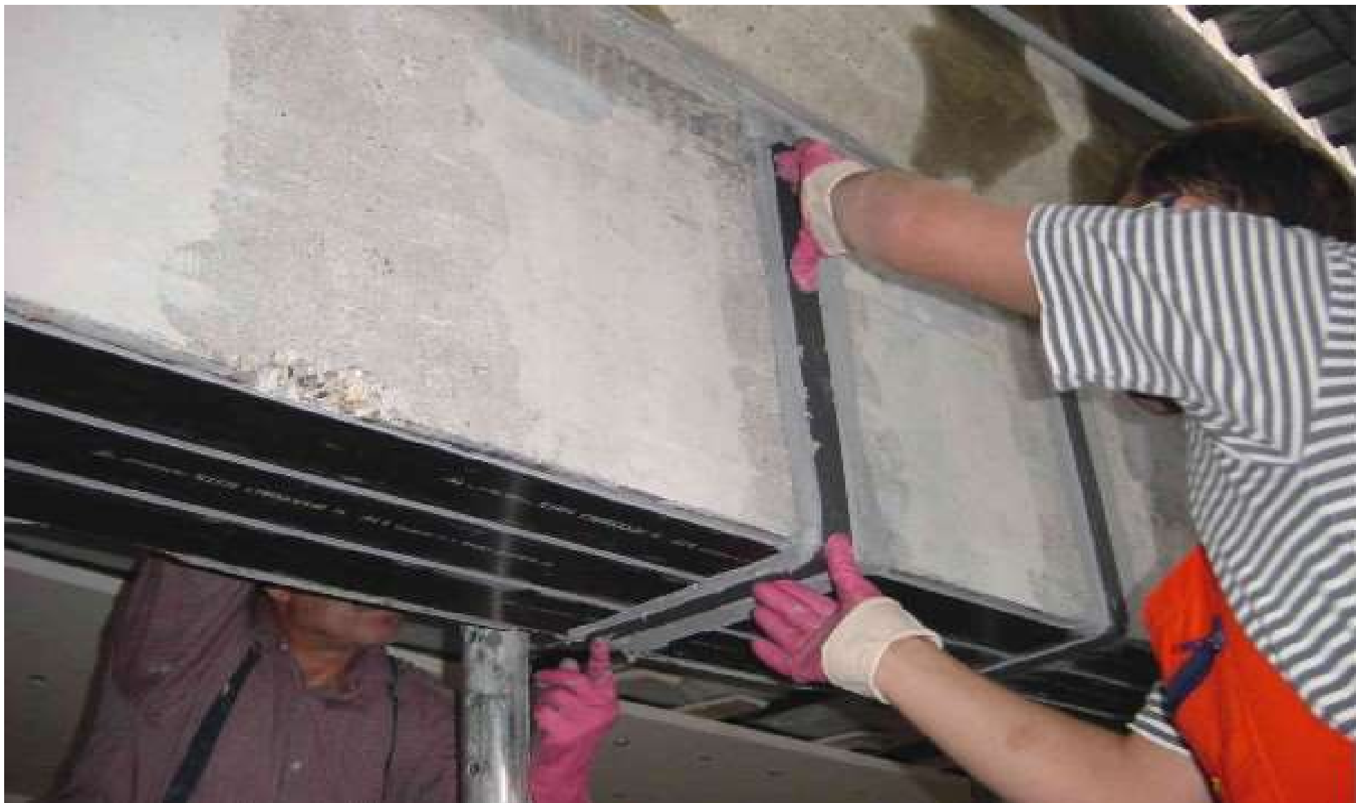
Installation of prefabricated CFRP L-shaped plates (shear strengthening) over existing CFRP strips (flexural strengthening)
