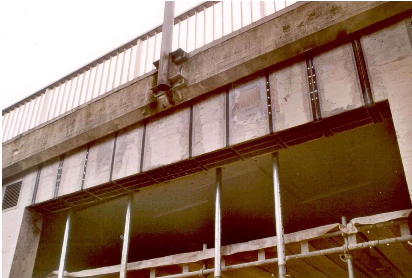
Externally Bonded FRP: Shear Strengthening
