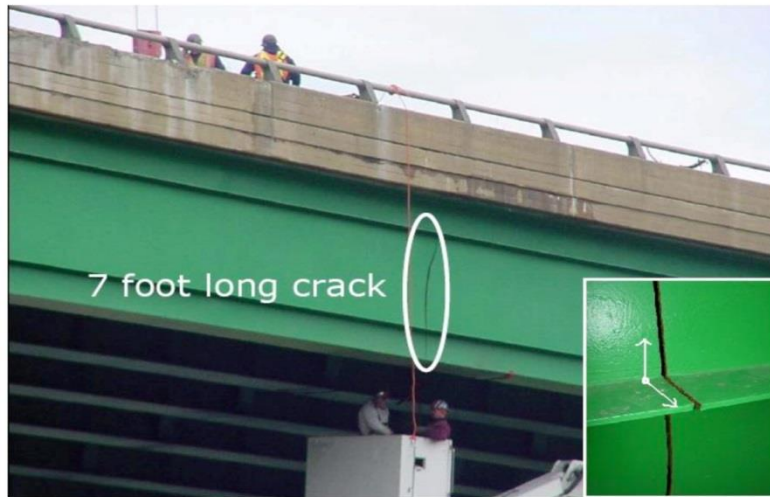
Chajes et al. „Fracture: Field testing of the I-95 bridge.“ In Third Annual Bridge Workshop: Fatigue and Fracture; Center of Innovative Bridge Engineering: Ames, IA,USA, 2004
