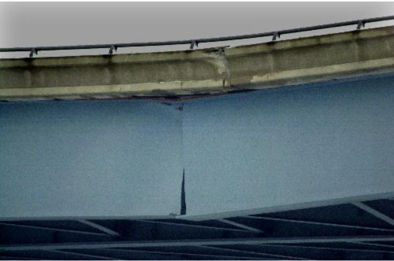
Daniel Hoan Memorial Bridge, Milwaukee, Wisconsin, Failure on the 13th of December 2000
