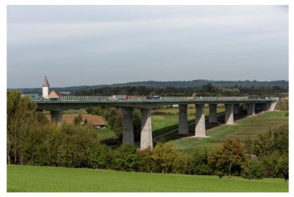
Bridge built 2001 no deviations from standards like concrete cover or concrete quality. Exposed to deicing salts
