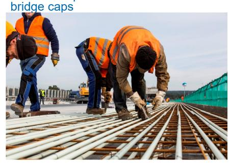
Longitudinal bars in FRP Perpendicular bars with more concrete cover still in steel
