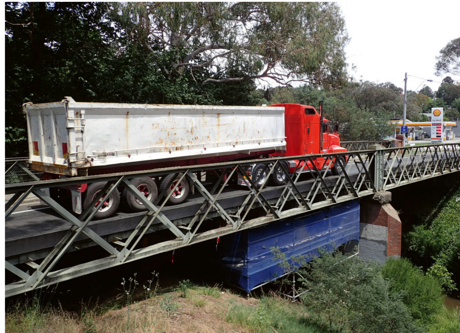
Diamond Creek Bridge near Melbourne was reinforced with CFRP strips in 2018 and, once the work was complete, its durability was tested with a 42-ton truck.
